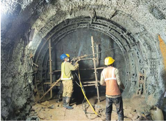
» Priority Sewer Tunnel Phase-I (PST-1) Project, Mumbai
