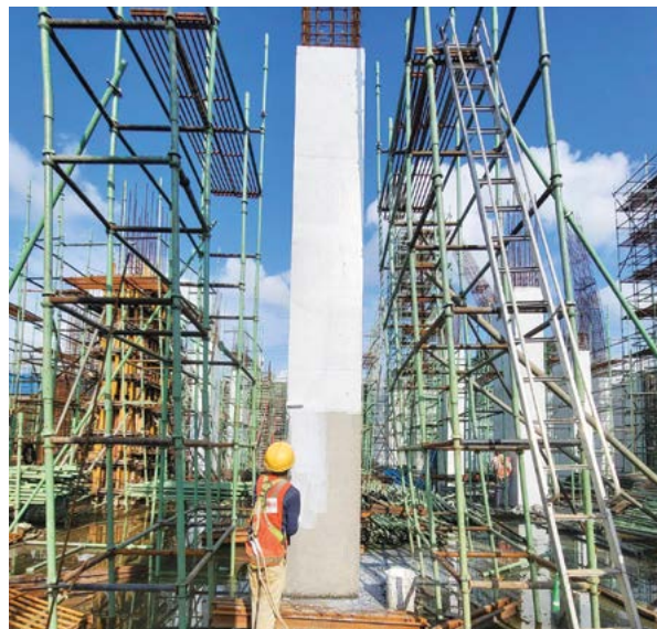
» Acrylic-based curing compound application
