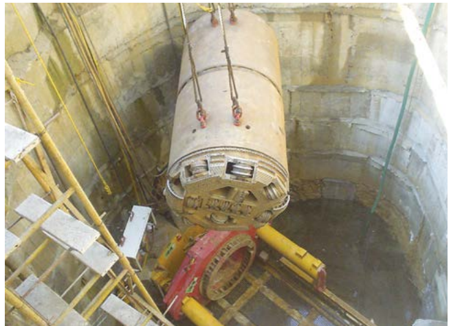
» Microtunnelling Project, Mumbai
