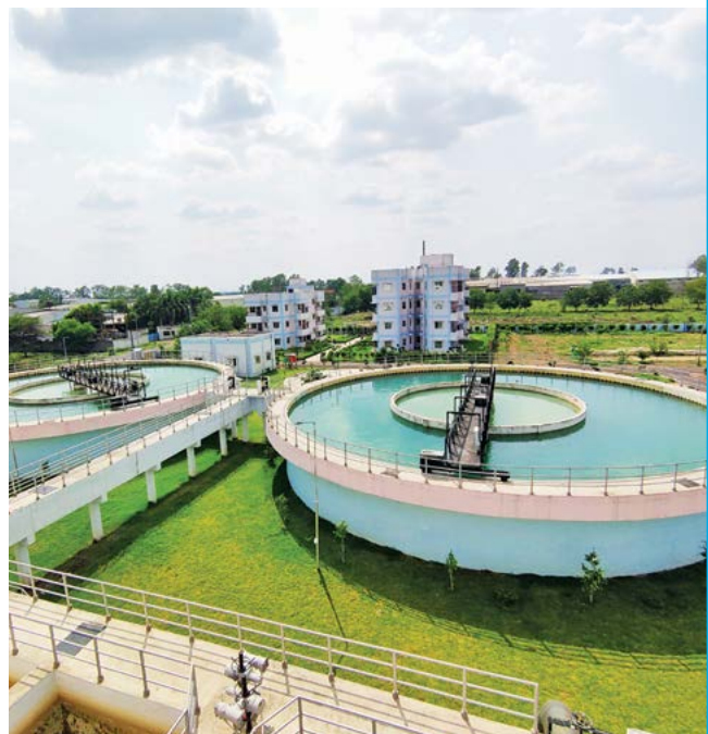
» Dewas Water Project, Madhya Pradesh
